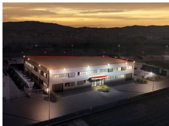
Figura 2 – Data Center IT2
