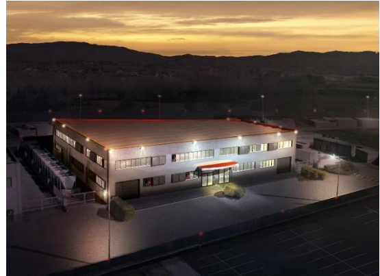
Figura 2 – Data Center IT2
